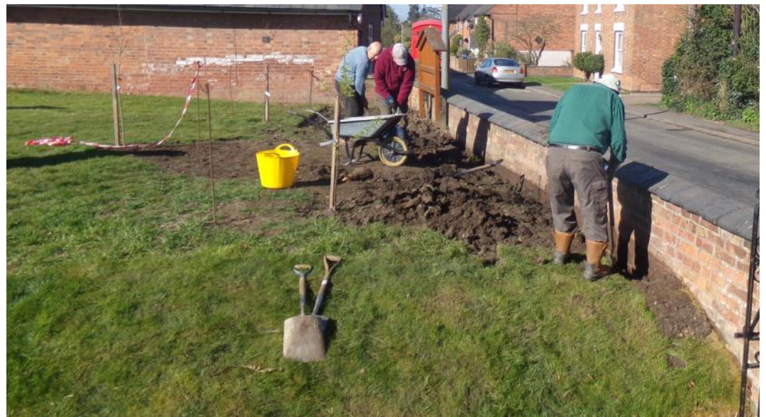
Installing drainage behind churchyard wall
